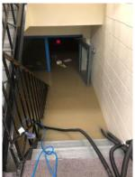
Mr. Franczyk and I arrived approximately 15 minutes after the flooding was noticed and there was already more than four inches of water covering the entire footprint of the lower level. Water could be seen gushing up from a trap door that leads to a crawl space under the lower level floor. As we watched, the water level continued to rise at a noticeable rate. Calls were
